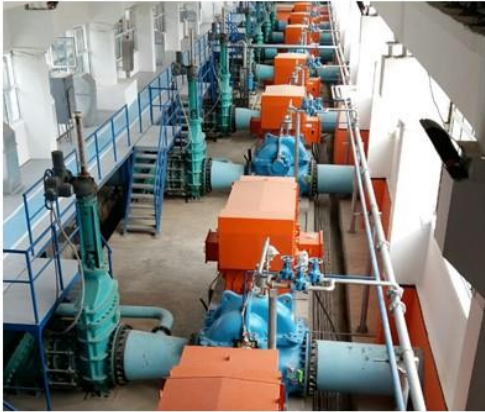
Bulokboshi Pumping Station
